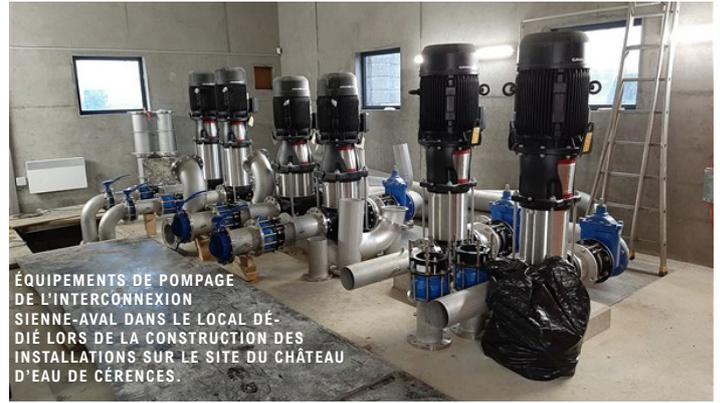
ÉQUIPEMENTS DE POMPAGE DE L'INTERCONNEXION SIENNE-AVAL DANS LE LOCAL DÉDIÉ LORS DE LA CONSTRUCTION DES INSTALLATIONS SUR LE SITE DU CHÂTEAU D'EAU DE CÉRÈCES.
